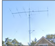
Fig. 3. The 14 MHz Yagi at WB7ABP had enough directivity to discriminate great circle and sidescatter headings.
